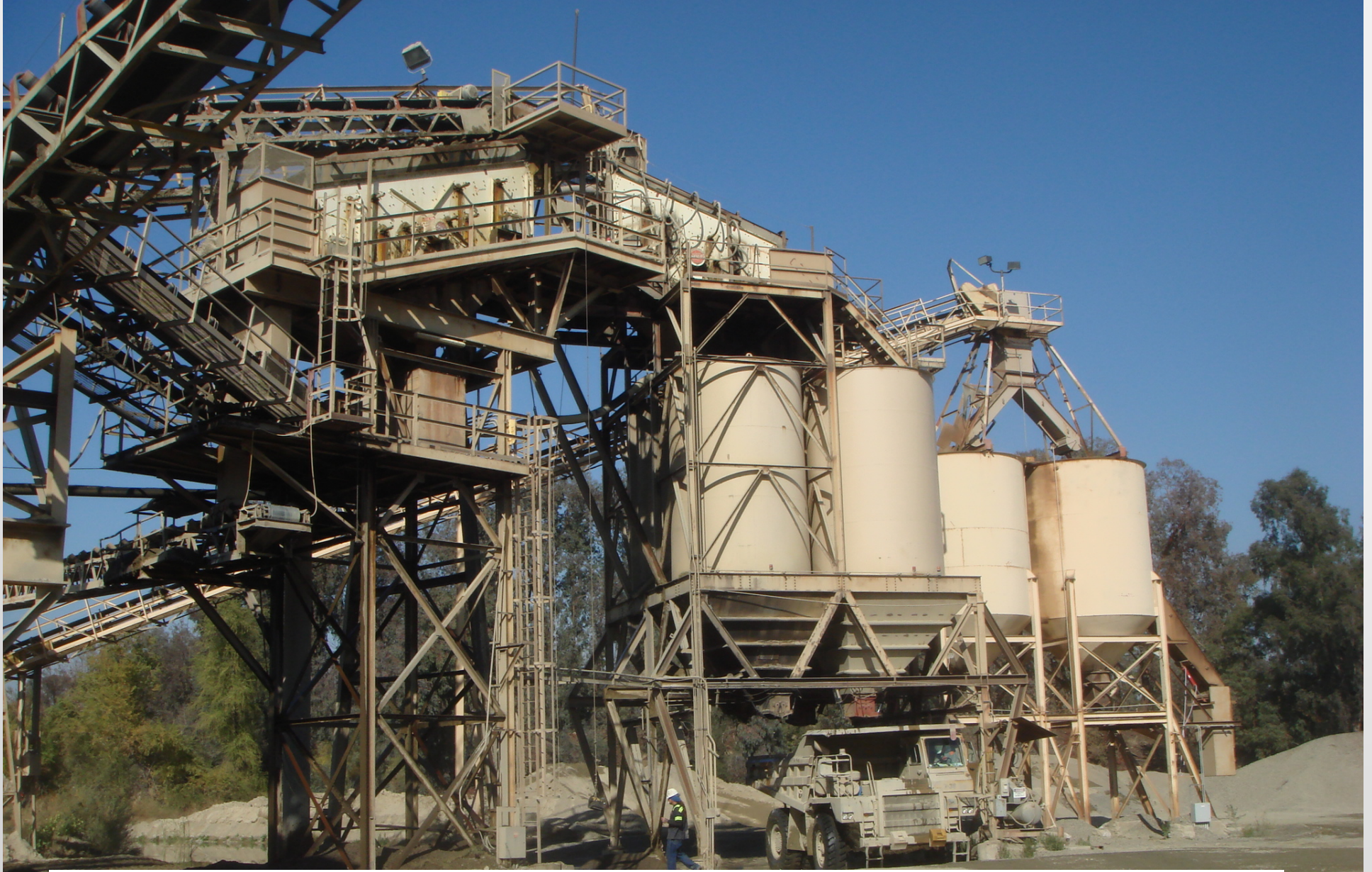
Wash Plant, Screens, & Truck Loadout
